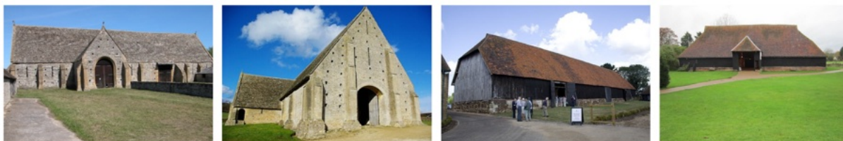
Middle Littleton Tithe Barn in Worcestershire (Philip Halling), Great Coxwell Barn in Oxfordshire (Andrew Mathewson), Harmondsworth Great Barn outside the Greater London (Prioryman, CC BY-SA 3.0, via Wikimedia Commons) and Barley Barn in Essex (Colin D Brooking, CC BY-SA 2.0, via Wikimedia Commons)
